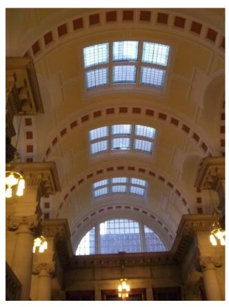
As part of the contract we carefully photographed each panel before dismantling and made careful note of any glass that needed to be replaced. Having supplied samples for approval prior to starting the work, we were able to get on with the careful restoration of the leaded lights bringing them back to their former glory.
